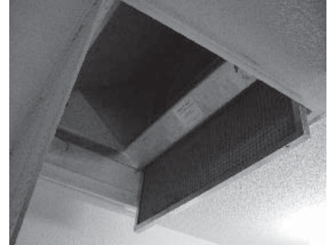
The filter slides vertically in and out of the filter slot.
