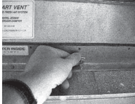
Turning thumb screws 180° to open filter door.
